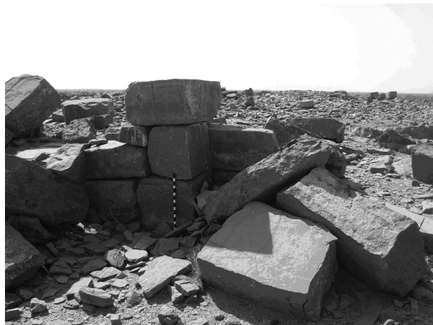
FIGURE 6. The offset in the east wall of Structure 1 at al-Khashbah.
