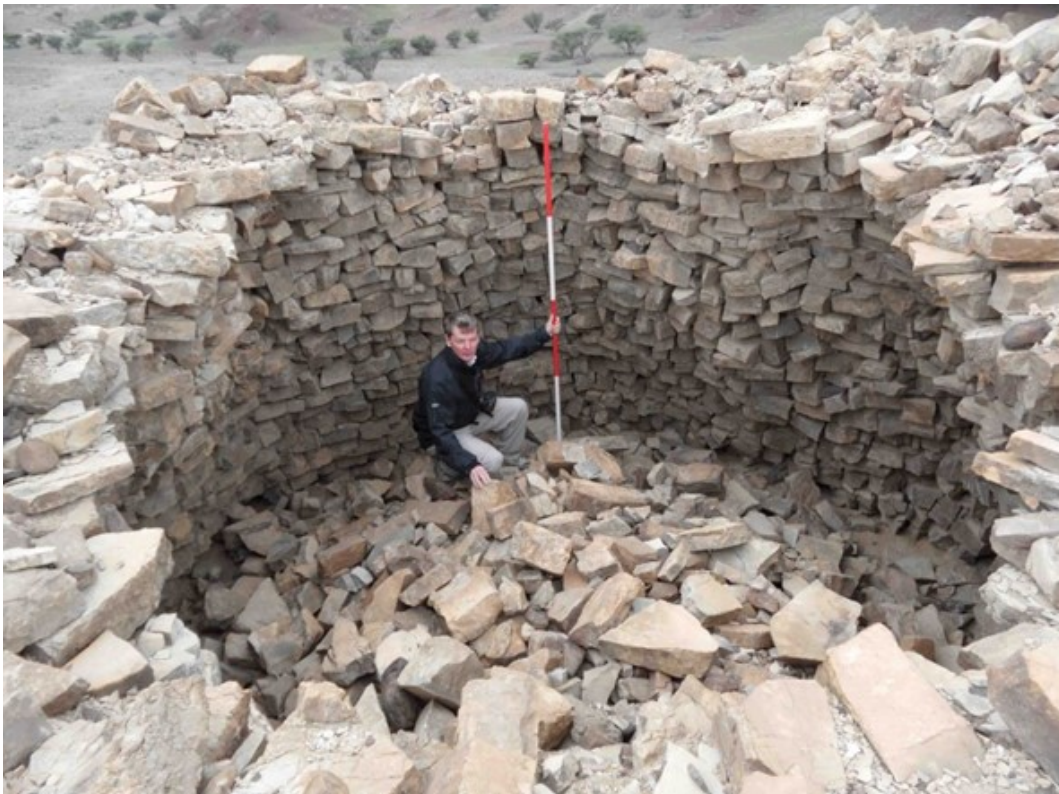
Fig. 50: View of the interior of the larger burial cairn showing the size of the corbelled chamber – which is clearly in imminent danger of collapse.
