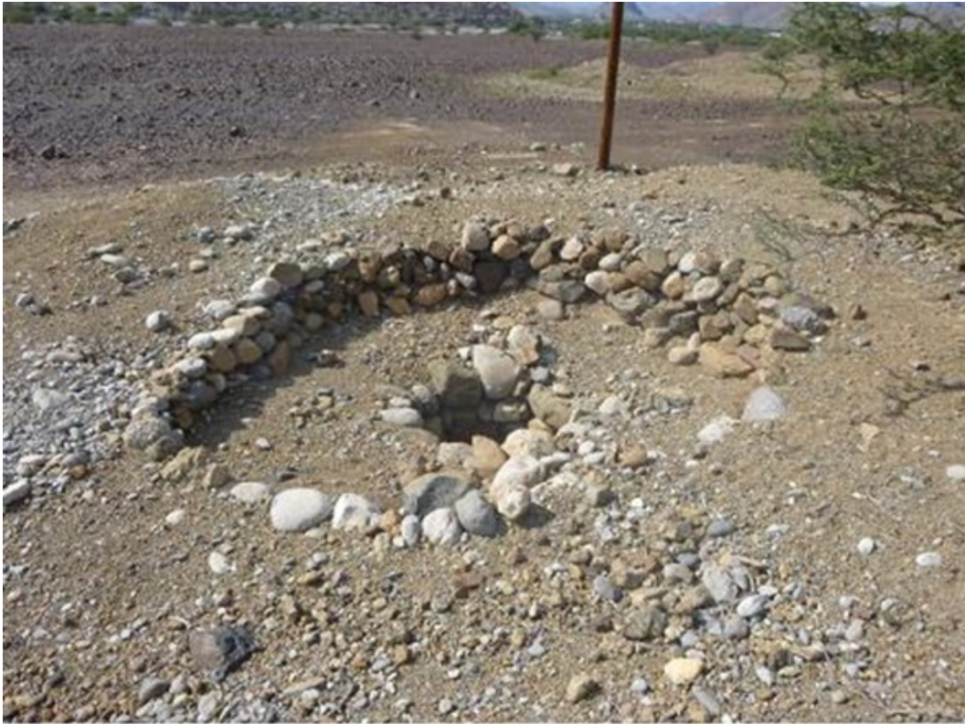
Fig. 75: A stone-reinforced up-cast mound around a falaj shaft .
