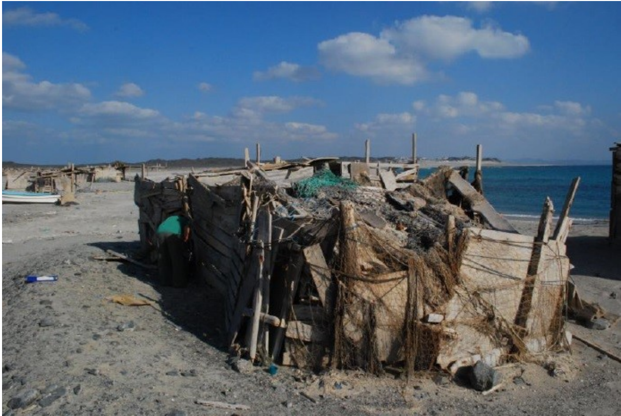
Figure (26) one of huts recorded at Haql.
