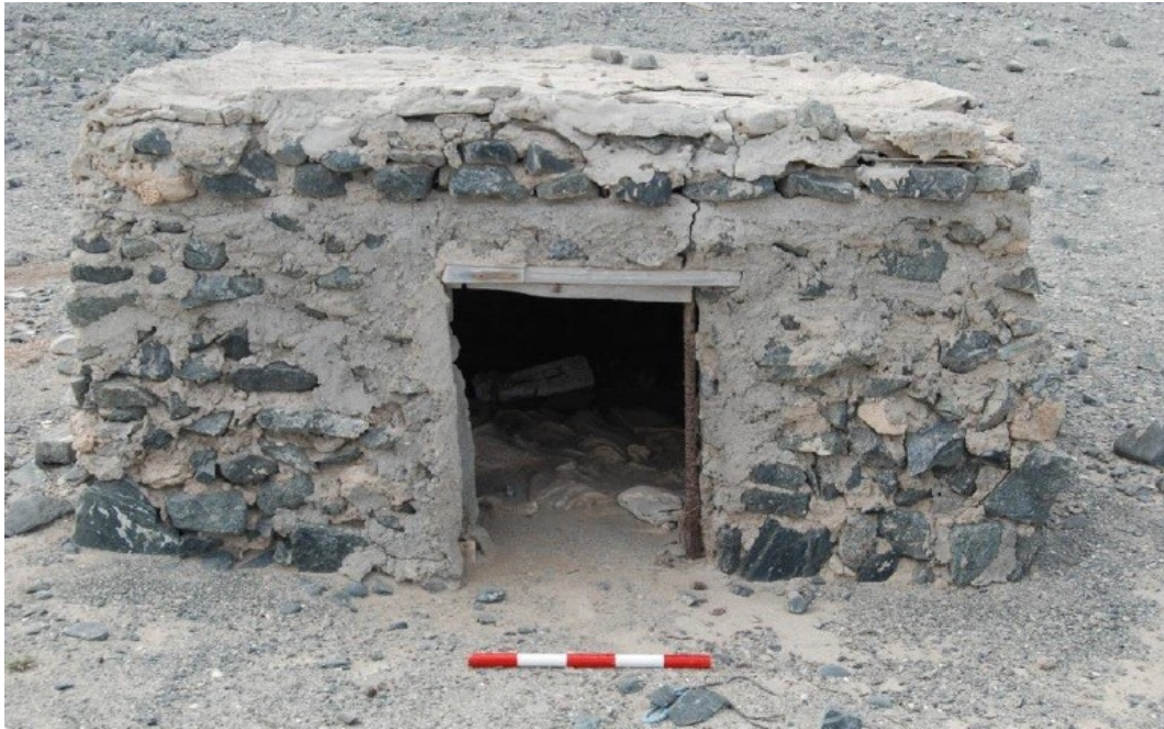
Figure (29) one of the two small stone built huts used for storing salted fish at Haql.
